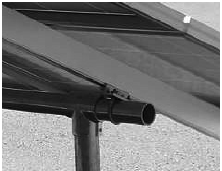
Attach Pipe Mount to Rail
