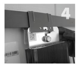
Slide this assembly onto the module frame with the bracket behind the module frame, the module level electronic mounting bracket in front of the module frame, and the bracket clamp in front of the module level electronic mounting bracket. Slide the assembly up and to the left to engage cap screw into bracket clamp slot.
