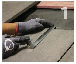
Determine the tile that the mount will be installed on. Remove the tile or tiles from the course immediately above that tile. Hook the top clamp over the top edge of the tile.
