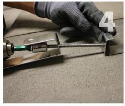
Insert the 4" tap bolt through the slot on the bottom clamp and into the threaded hole on the end of the top clamp. Use a 7/16" socket wrench to thread the screw.
