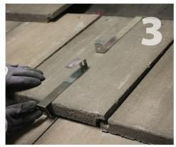
Slightly lift the bottom of the tile and slide the bottom clamp over the bottom edge of tile.
