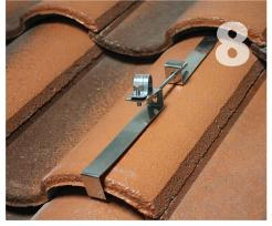
is the same. Make sure that the conduit mount is installed onto the crown (high point) of the tile not in the valley.
