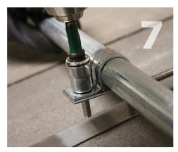
Insert conduit and use a 7/16" socket to tighten down the pipe clamp.
