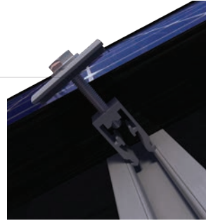
Image 6.4.1 Inner module installation step 1
