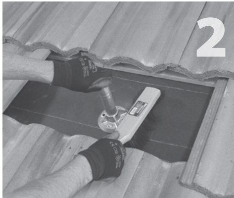
Clean away dust and debris around QBase.
