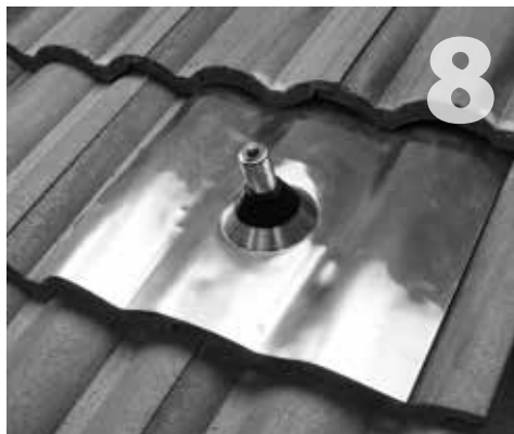
Install the 18"x 18" flashing (item 6). Pre-bend the flashing to follow the contour of the tile if curved. Apply sealant where post and flashing meet, and install EPDM counter flashing collar (item 7). Be sure to seal off the post from weather exposure with the racking hardware (items 8-11) in the interim before racks are installed.
