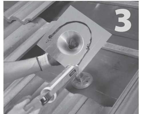
Apply a bead of sealant in the shape of an upside down U on the back side of the subflashing.
