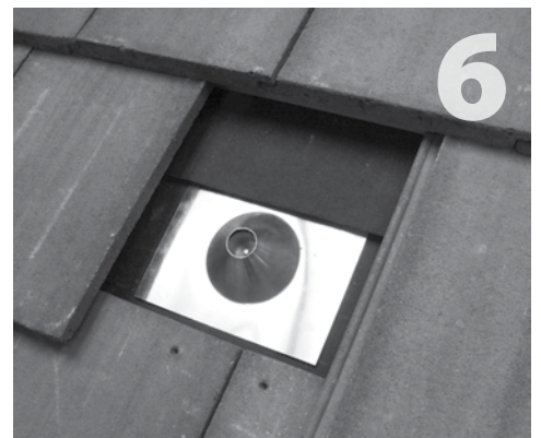
Take care to do a quality installation. When using the paper method, slide subflashing under felt overlap or cut an additional piece of felt paper 18" wide to slide under the course above, and over the primary flashing of the mount. This is essential for proper waterproofing.
