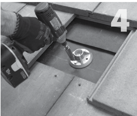
Align QBase (item 1) over rafter center and drill two 7/32" pilot holes. Fill pilot holes with sealant compatible with roofing material. Place grade-8 cap screw (item 2) under QBase in hex slot, threads pointing up. Lag QBase into rafter through pilot holes.
