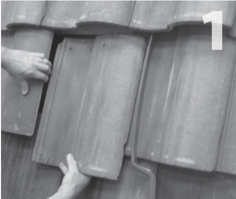
Remove tile at selected location of mount.
