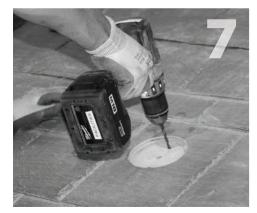
Using QBase (item 2) as a guide, align two clearance holes vertically with the center of the rafter. Mark the center of these 2 holes. Drill 7/32" pilot hole at each of the 2 marks. Hold drill square to rafter. Do not use QBase as a drill guide.
