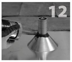
Apply a bead of sealant around the area where the cone flashing meets the post.
