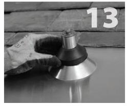
Install the EPDM rubber counter flashing over the post, and attach all the remaining hardware (items 7-10) on top of the post for safekeeping until the racking is ready to install.
