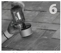
the lower portion of slate with a slate ripper, then pilot hole drilled in step 3, drill through the existing
