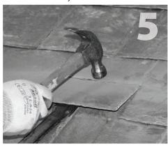
To remove the slate below the score, slightly lift Using a 4" diameter diamond hole saw and the gently but firmly tap the top piece with a hammer. slate. The lower piece should break off cleanly.
