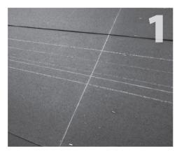
Lay out your array over the felt paper using a chalk Using the QBase as a guide, mark pilot hole line to mark rafter centers and the rail location centers.
