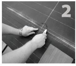
location for drilling. If roof is already felted, cut a section in the topmost layer for the QBase, so that the shakes underneath can still slip under the felt.
