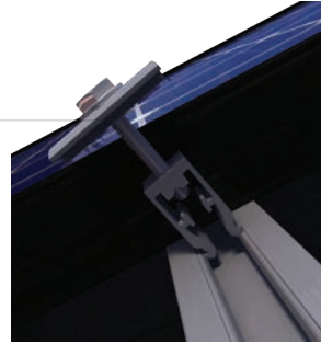
Image 6.4.1 Inner module installation step 1
