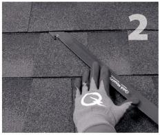
Carefully lift composition roof shingle with roofing bar, just above placement of mount. Remove nails as required and backfill holes with aproved sealant. See "Proper Flashing Placement" on next page.
