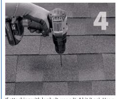
If attaching with lag bolt use a 7/32" bit (Lag). Use a 1/32" bit (ST) for attaching with the structural screw. Drill pilot hole into roof and rafter, taking care to drill square to the roof. Do not use mount as a drill guide. Drill a 2" deep hole into rafter.
